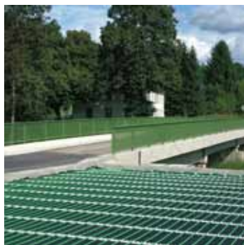
Open space heating
