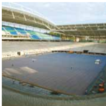
Undersoil pitch heating
